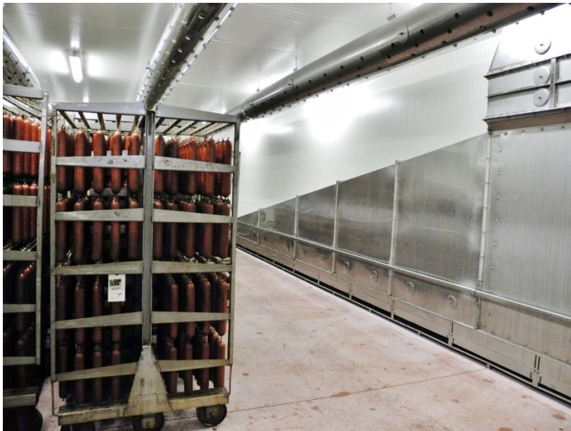
Fig. 2: Illustrative photo: Not only the inlet of air-conditioned air but also its outlet play a role for a uniform and efficient process of sausage drying. The picture shows installations that extract air from the chamber into the air conditioning unit located on the right wall, manufacturer MAUTING KMD CrossFlow.
