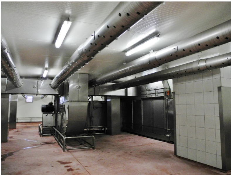
Fig. 1: Illustrative photo: ripening climatic chamber MAUTING KMD CrossFlow. The aim of the designers and manufacturers of air-conditioned chambers is to ensure intense water loss during the drying of sausages without causing a ring formation or other defects. The uniformity of drying throughout the chamber is also important.
